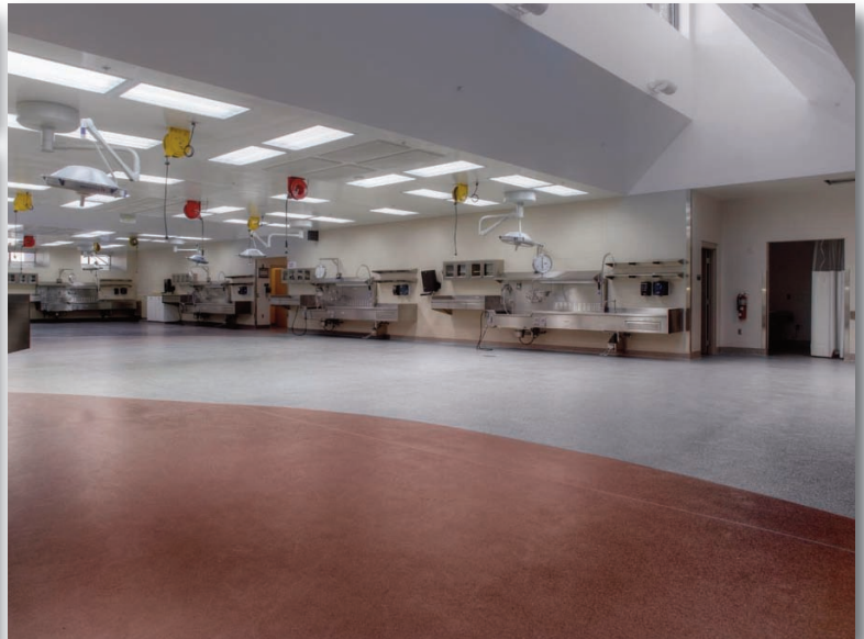
Stonblend GSI-G incorporates recycled glass aggregate into the floor surface, creating a sustainable, durable floor for the autopsy area.
