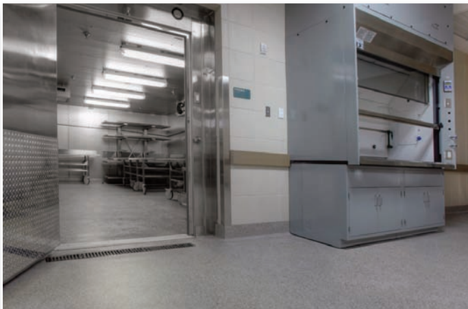
In the coolers, Stontec TRF floors are reliable, despite temperature extremes and heavy traffic.
