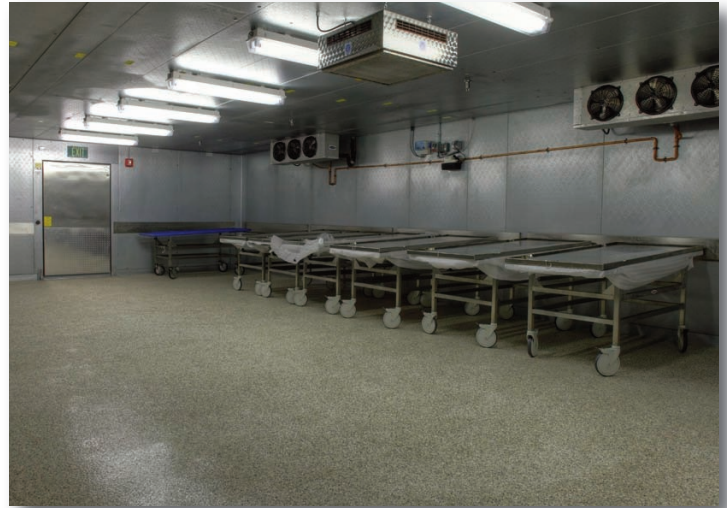
Stonhard's Stontec TRF and Stonblend GSI-G systems are hard-working, chemical-resistant, textured for slip-resistance and easy to clean at the District Nine Medical Examiner's Office.
