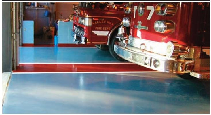
Firehouse floors have a Stonhard epoxy system with a urethane coating that is safe, improves cleanability, stain resistance and UV resistance while providing a glossy, sleek finish.
